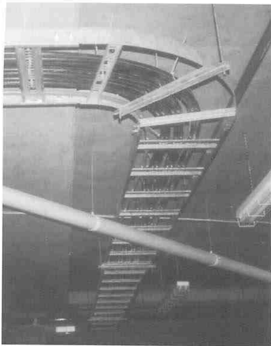
Fig. 10.1(c) Non-metallic sheathed fire-retardant cable installation
