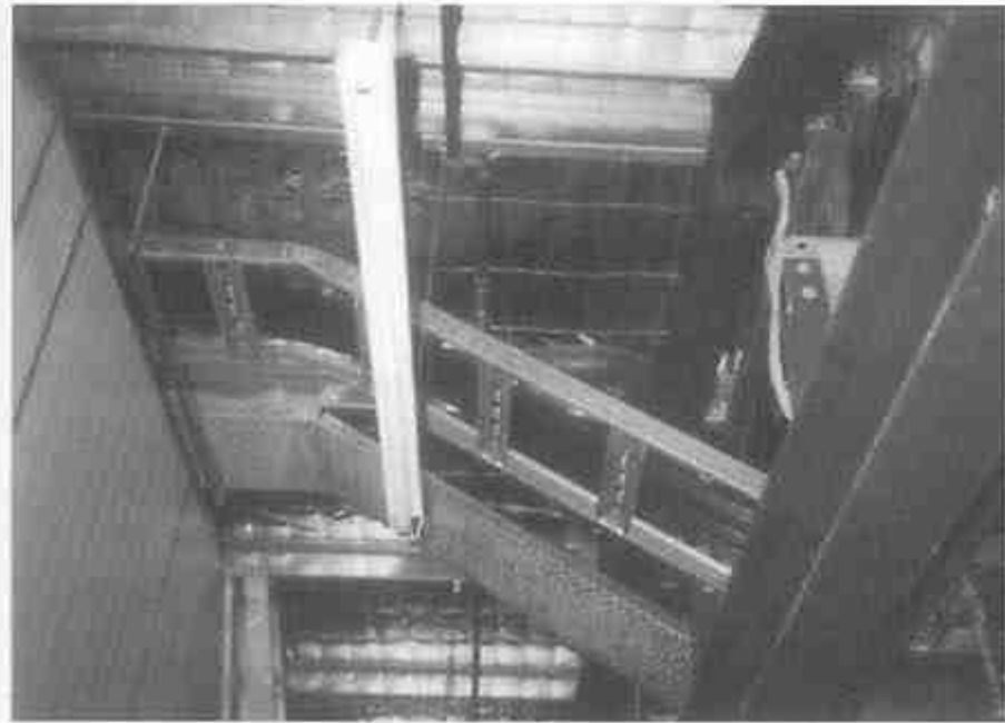
Fig. 7.14 Perforated-tray cable support (background) and ladder support (foreground) OLEX CABLES
