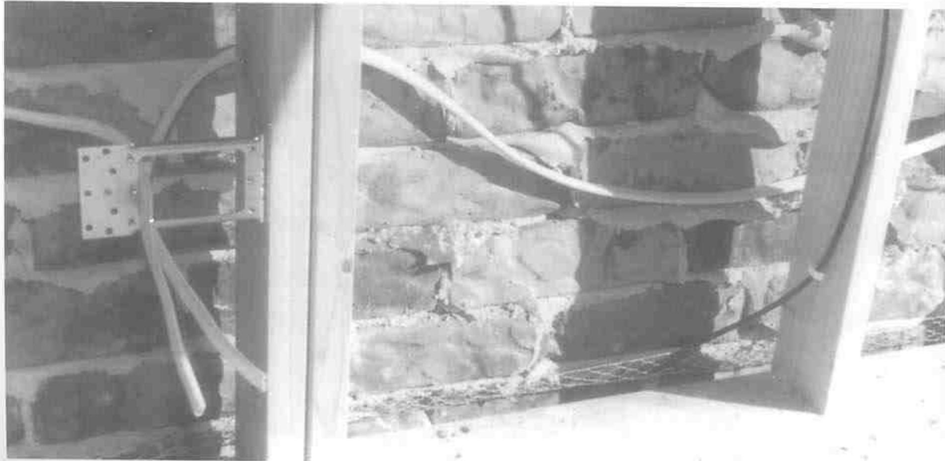
Fig. 8.9 Cables supported on wall ties (not permitted in Victoria)
