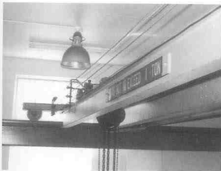
Fig. 7.1 Crane collector wires
