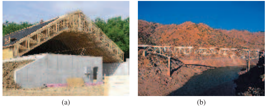
Figure 6.1. Examples of truss structures. (a) The roof of this highway maintenance building under construction uses 124 identical wooden roof trusses with 16 in. spacing. (b) Mores Creek bridge over Lucky Peak Reservoir near Boise, Idaho.
