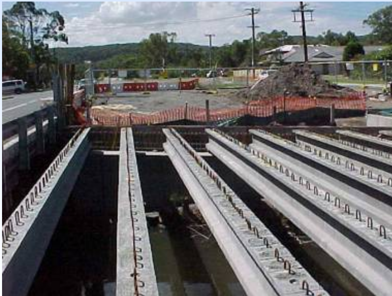
Ductal beams in place
